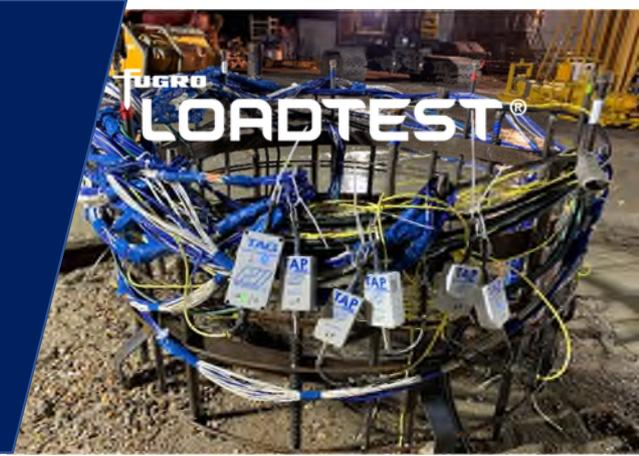
Fugro LOADTEST has been performing Thermal Integrity Profiling on both preliminary and working foundation elements for many years.
